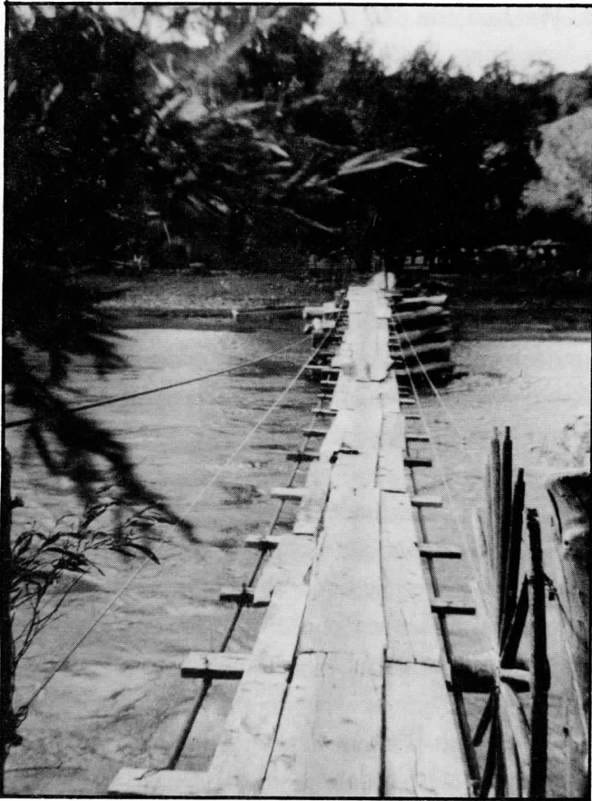
Roybal's suspension bridge
